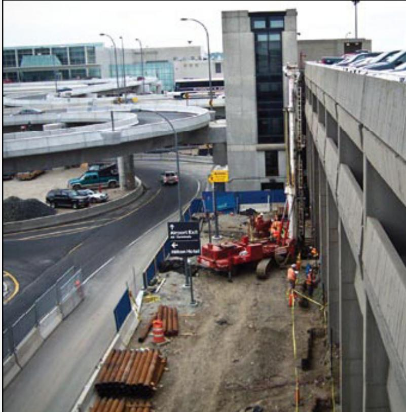
Micro piles are a system of soil inclusions using steel bar reinforcement and cement grout combinations with or without steel casing that are mainly used as friction piles to take tensile or compressive loads.
