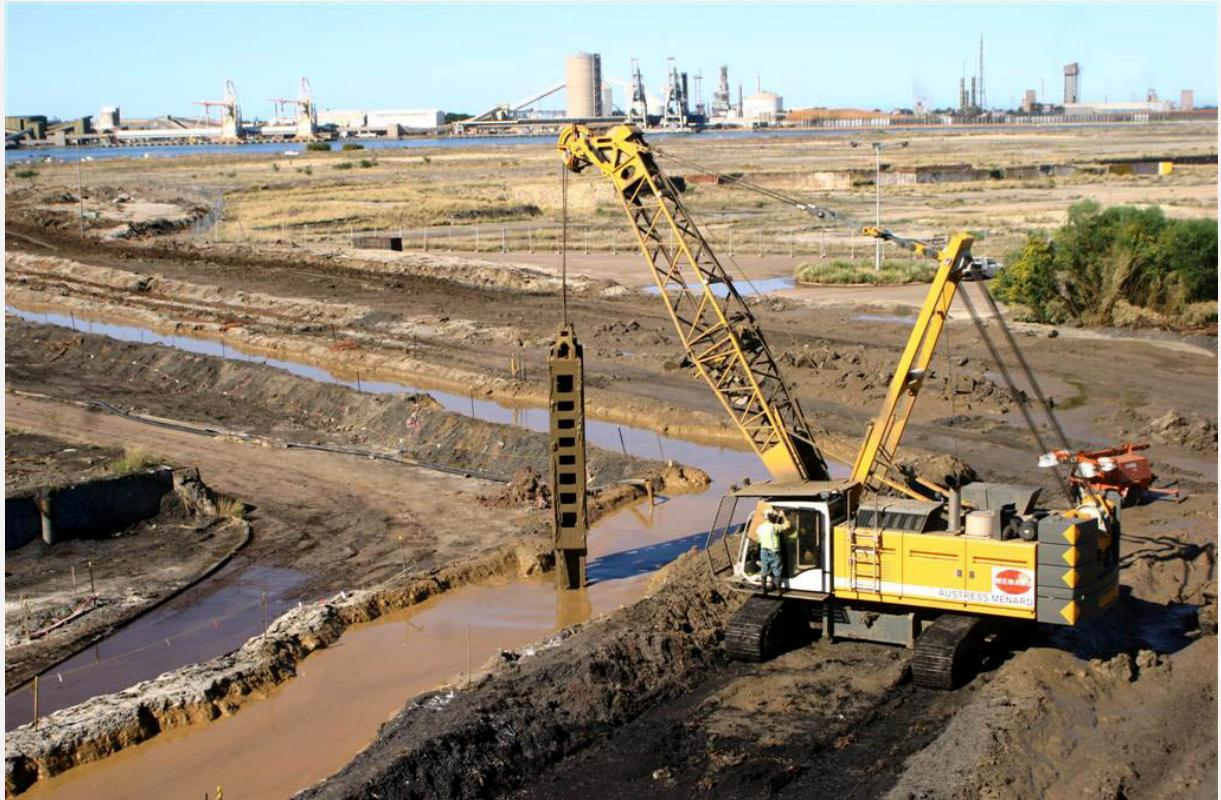
Slurry walls are an effective way for creating a cut-off barrier and preventing the flow of water. They are frequently used in dams and contaminated sites.
