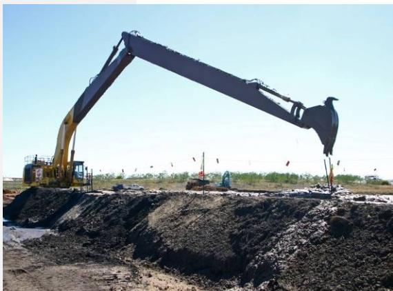
A slurry wall as deep as 50 m and 1500 m long was required to block the flow of water from the former Newcastle Steelworks site in Mayfield, NSW into Hunter River.
