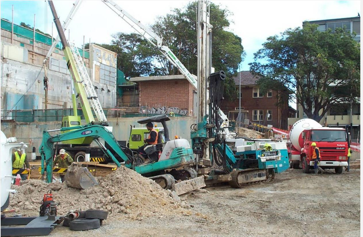
Cavity grouting of macro voids with bulk materials is a safe technique for ensuring that structures built on the ground will not be influenced by the sudden collapse of the cavity.
