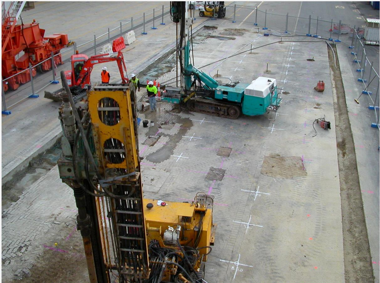
Compaction Grouting provides an appropriate method of improving the engineering properties, density, and shear strength of loose soils.
