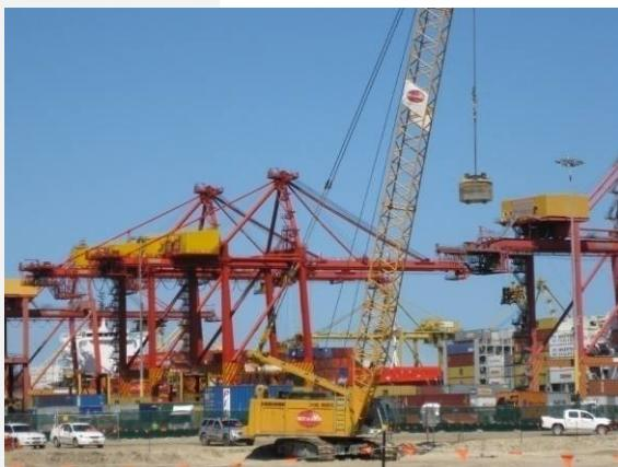
Dynamic Compaction, proven to be the most affordable and highest production ground improvement method has been used for the treatment of the loose reclaimed soil at Sydney's Port Botany.
