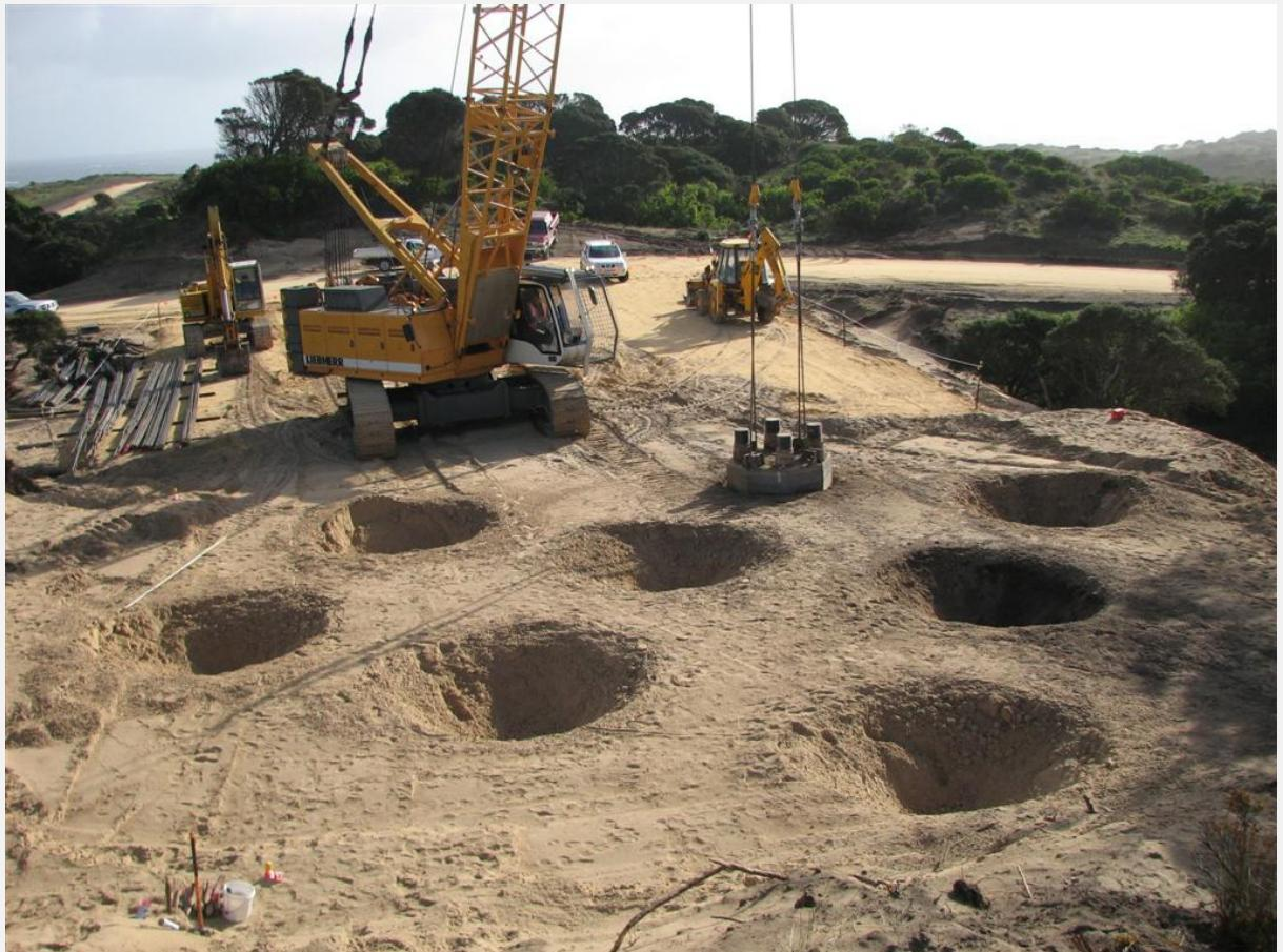
Dynamic Compaction is one of the techniques invented by Louis Menard for compacting soils to great depths. This technique is applicable to all clean granular soils, and to dry, partially saturated and saturated soils with substantial amounts of fines.
