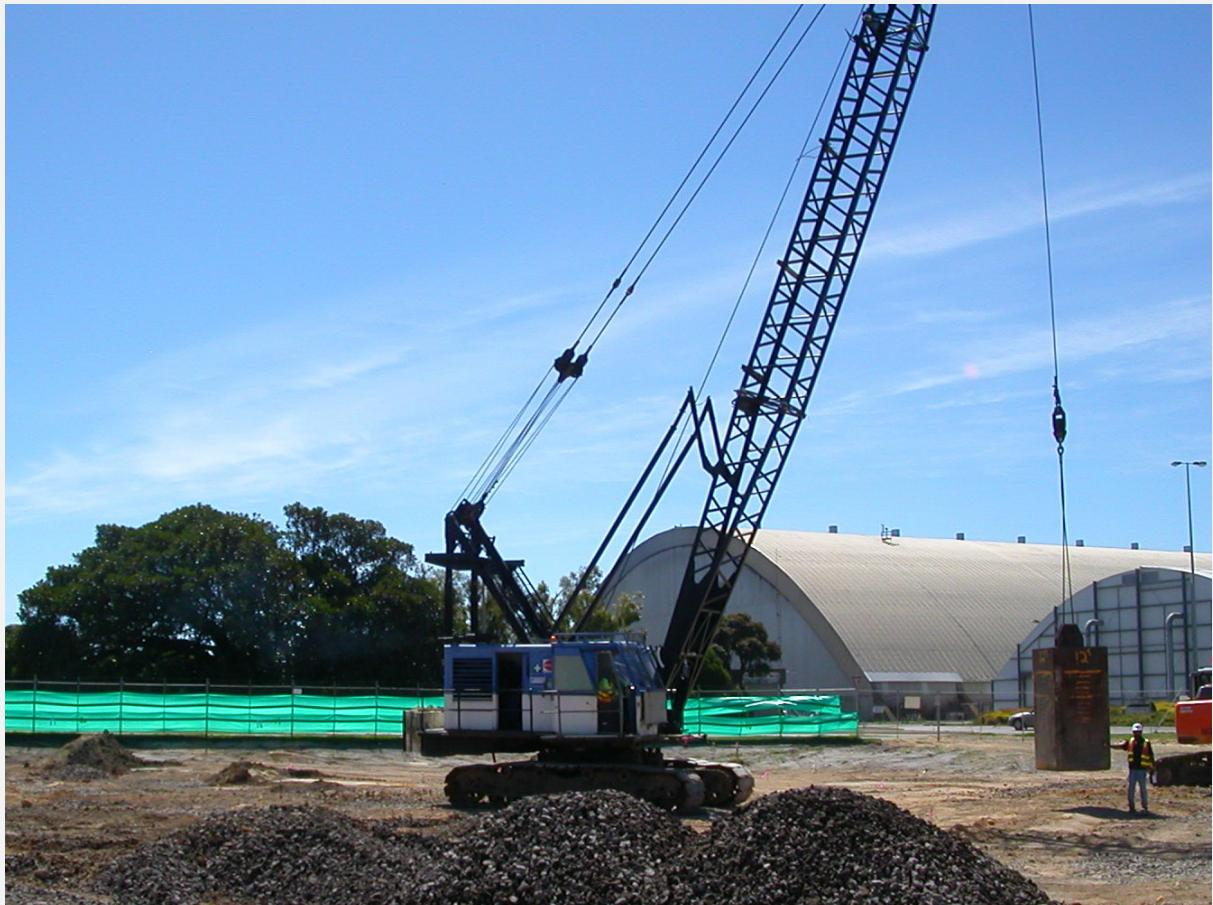
Dynamic Replacement is one of the techniques invented by Louis Menard for improving the strength of saturated soft cohesive or organic soils. This technique is applicable to all clean granular soils, and to dry, partially saturated and saturated soils with substantial amounts of fines.
