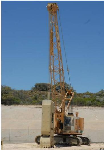
As part of the intake, outfall and TBM launch chambers of this project 38 diaphragm wall panels and 28 barrettes, each 25 m deep, were constructed. Total wall length was 250 m.
