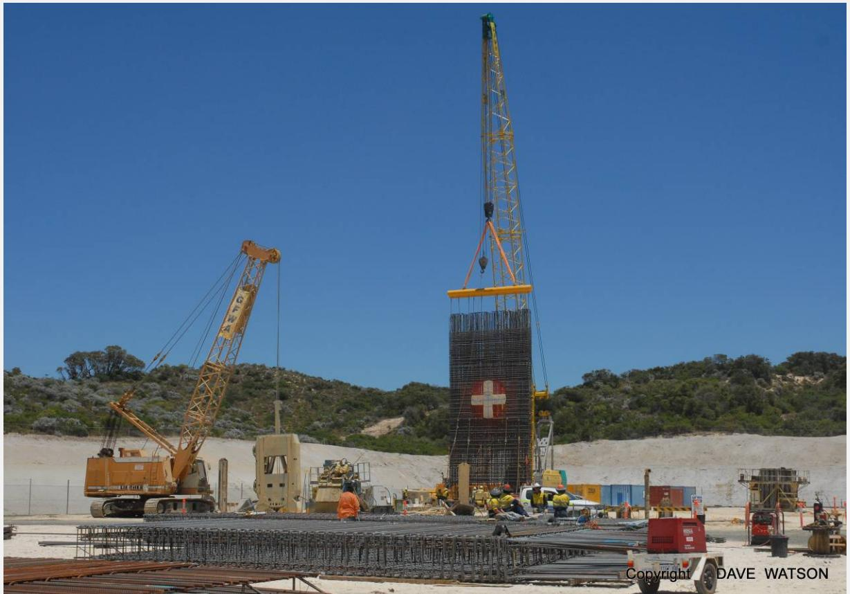
The principle concept of a Diaphragm Wall is to construct a retaining wall within a slot excavated in the ground. Once completed the diaphragm wall can be used as a retaining wall for a multitude of applications, for example basement walls, earth retaining wall, water storage tank, cut off walls, etc.
