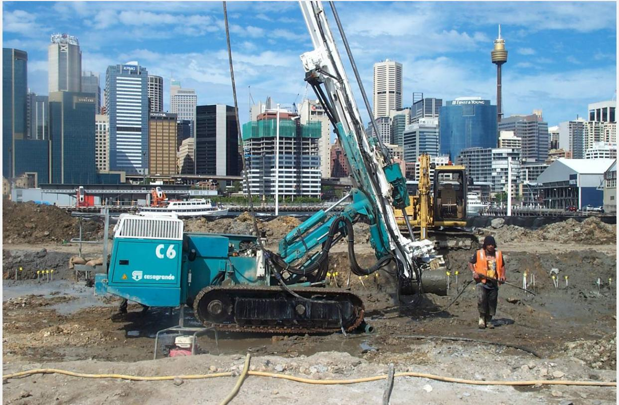
Jet Grouting is a very effective technique for minimizing ground settlements, stabilizing excavations or creating impervious surfaces.
