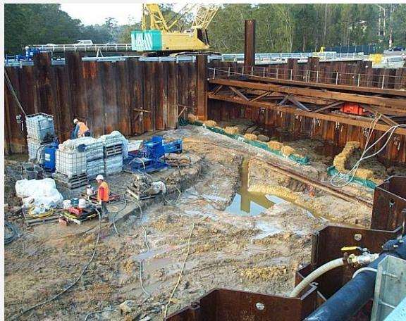
12,000 m<sup>3</sup> of micro fine and ultra fine cement grouts were pumped into the ground at the location of the cofferdam boundaries and the service facility basement at the Lane Cove River Tunnel of Parramatta Rail Link project that links Chatswood to Epping.
