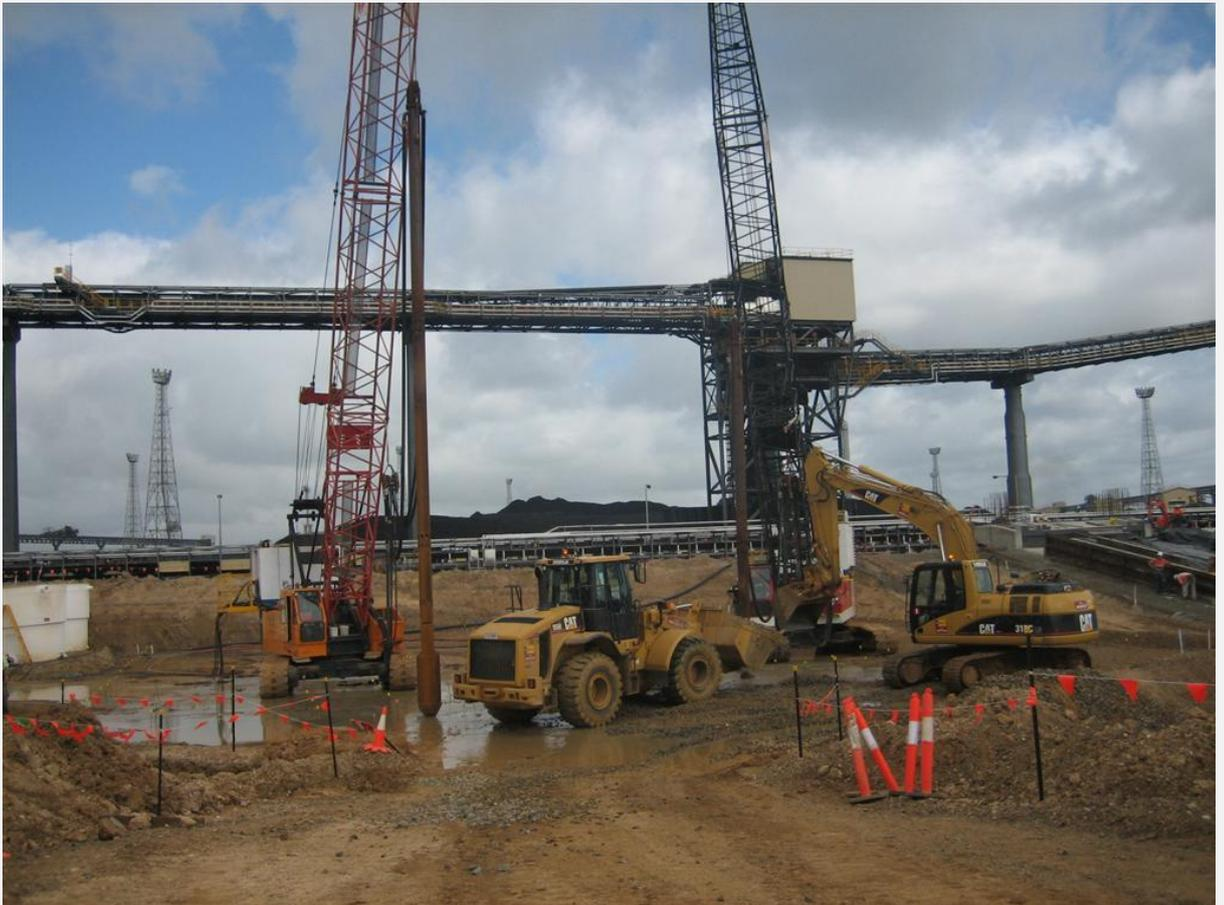
Vibro Replacement (Stone Columns) improves the strength of deep saturated cohesive soils using a vibroflot.
