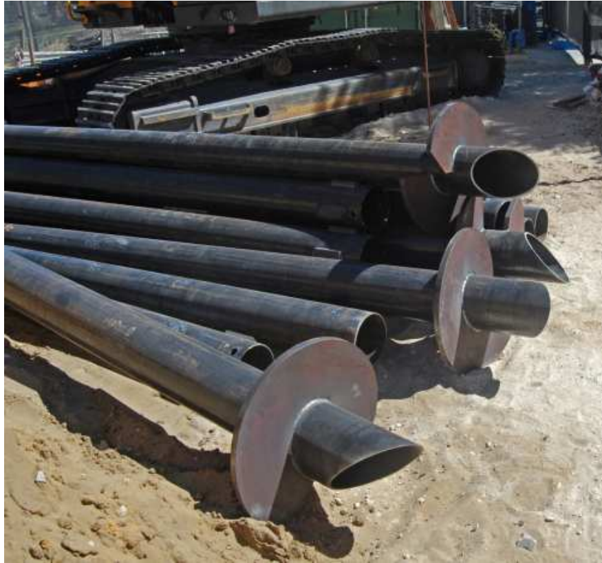
Helical shaped plates welded to the steel shafts of the screw piles
