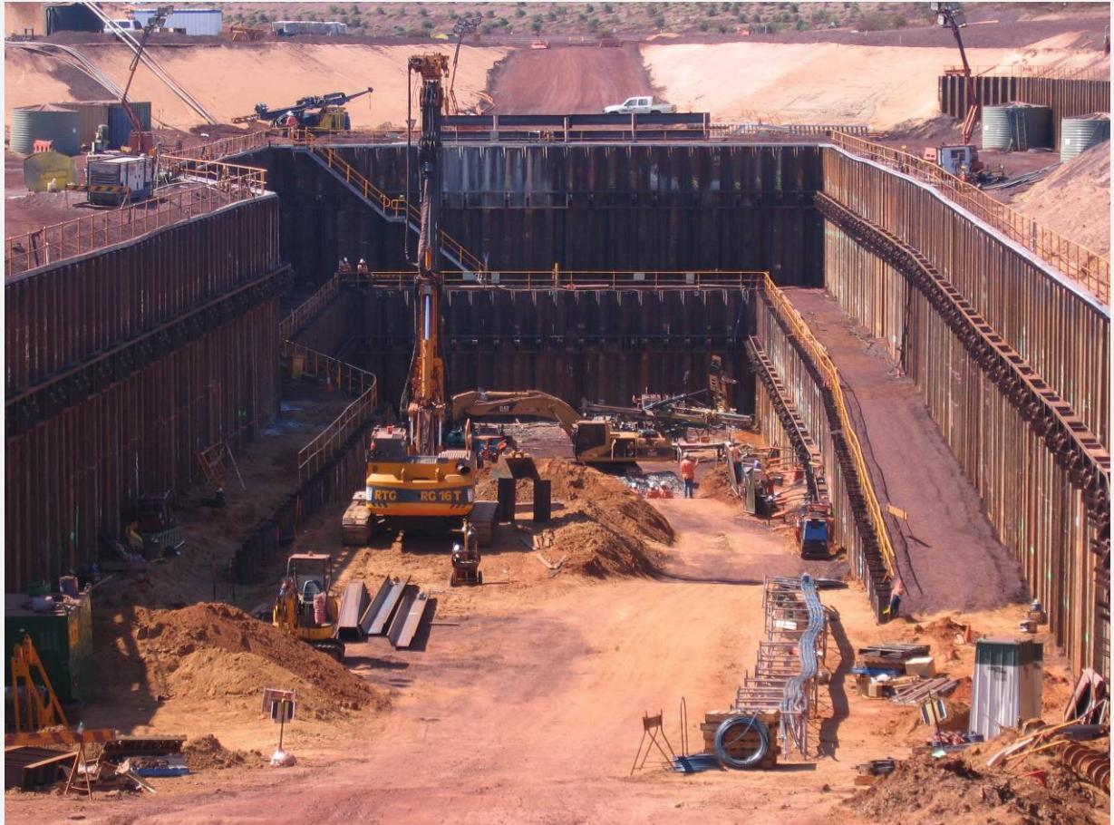
Sheet piling is an efficient and affordable wall system that can be used to retain the ground both in saturated and unsaturated conditions, inland, near shore and offshore, and for temporary or permanent retaining. In this system the sheets are driven into the ground to the desired depth, and thus construction of footings is avoided. External stability is made available by providing sufficient amounts of horizontal passive reaction or additional reaction using ground anchors.
