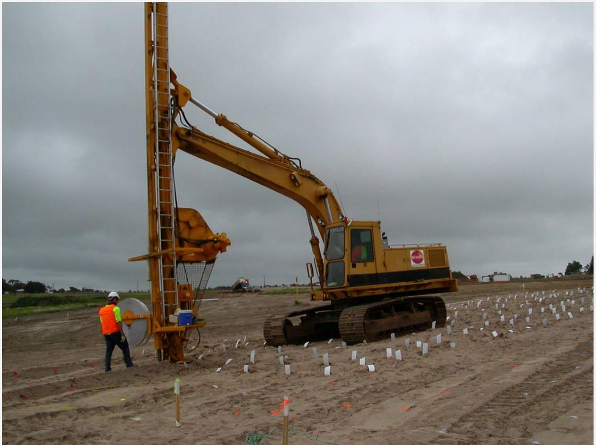
Vertical drainage can be used to accelerate the consolidation of impervious soft silts and clays. Prefabricated vertical drains (PVD) are flat or round flexible polymer tubes.
